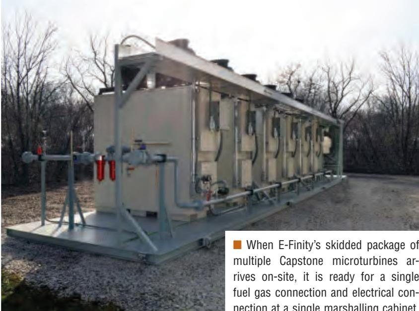
■ When E-Finity's skidded package of multiple Capstone microturbines arrives on-site, it is ready for a single fuel gas connection and electrical connection at a single marshalling cabinet, which can reduce installation time to just a few hours.
